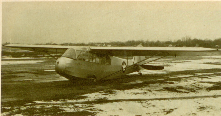
An odd J-3 variant for the Army was the TG-8. The original nose was cut off and a third seat was added in the new glider nose to maintain the balance. The object was to create a training glider that had the flight characteristics of the boxy cargo gliders that the students would fly later.
